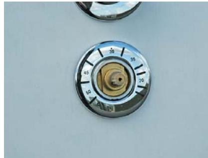
Remove the plastic temperature guard from the brass spline exposing the head of the core.
