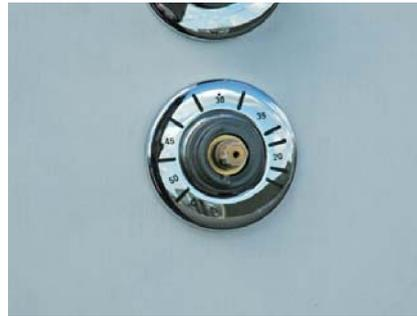
Remove the temperature selector knob. Remove the chrome coloured plug in the dial to allow access to the Alan grub screw inside. Loosen the dial until it removes easily.
